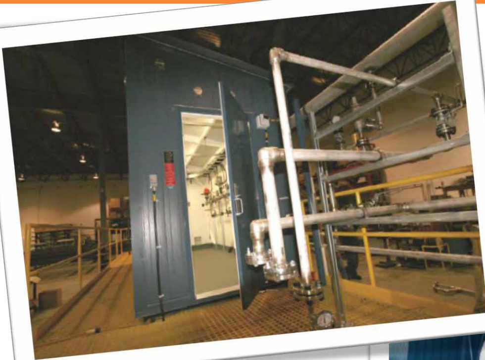
Liquid SO 2 Building
